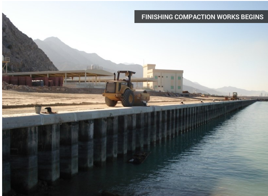
READY FINAL COMPACTION CONTINUES NOW THAT ALL SHEET PILES AND TIE RODS ARE INSTALLED
