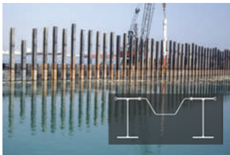
FUJAIRAH BREAKWATER BERTH, UAE
