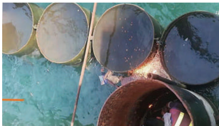
PORT REHABILITATION PROJECT, PHILIPPINES
