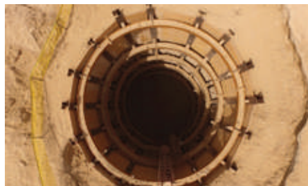
CIRCULAR COFFERDAM, UAE
