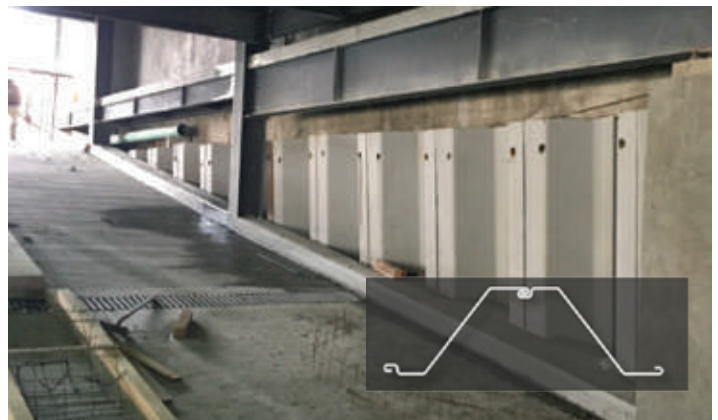
UNDERGROUND PARKING LOT, MEXICO
