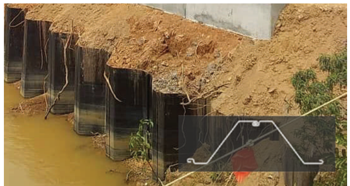
PAHANG BRIDGE ABUTMENT, MALAYSIA
