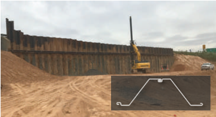
RETAINING WALL, VIRGINIA, USA
