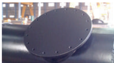
FENDER FLANGE CONNECTION
