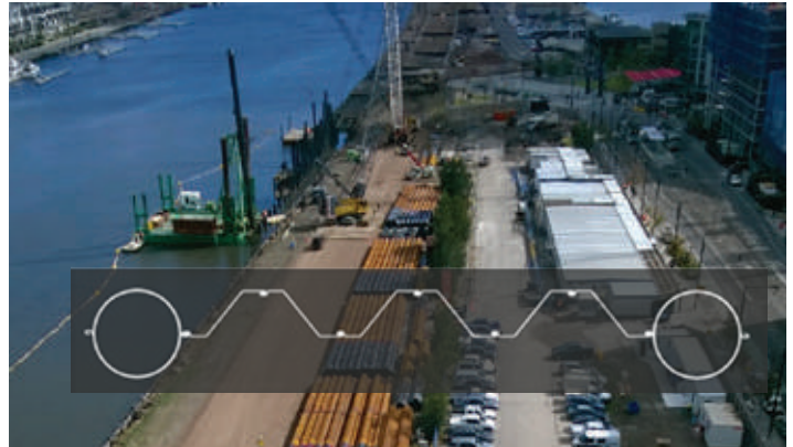
VICTORIA HARBOUR EXTENSION, AUSTRALIA
