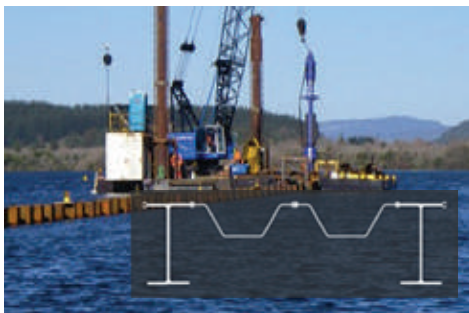
OHAU CHANNEL DIVERSION, NEW ZEALAND
