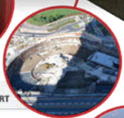
SHEET PILE PERMANENT BASEMENT WALL
