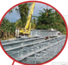
STEEL BRIDGE GIRDERS
