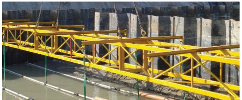
TIE ROD SPREADER BEAM
