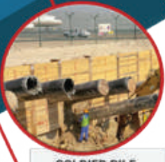
SOLDIER PILE & TIMBER LAGGING
