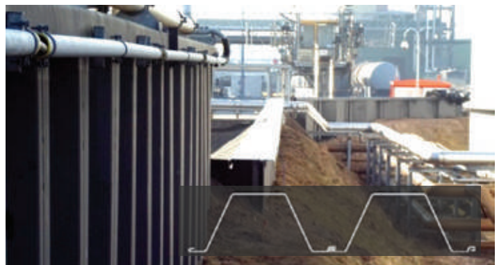
CONTAINMENT BARRIER, NETHERLANDS
