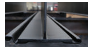
H PILE COLD FORMED INTERLOCK
